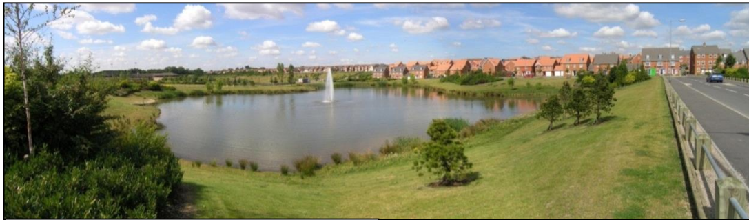
Sustainable Drainage Scheme Corby
